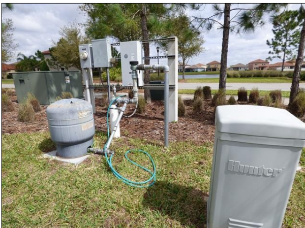
Irrigation System and Well
