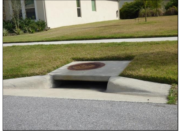
Stormwater Drainage Curb Inlet
