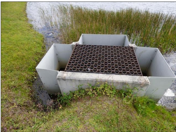
Stormwater Drainage Control Structure
